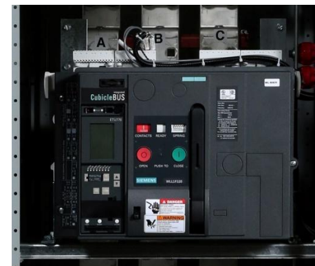
Fixed Circuit Breaker
